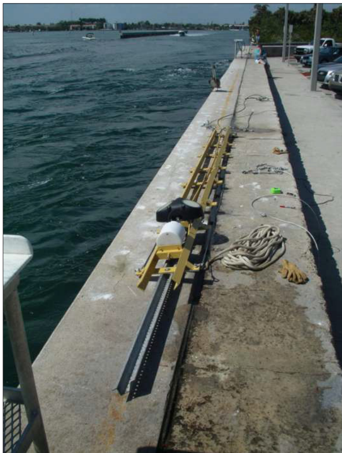
Figure 3. Aragonaut 500-kHz side-looking acoustical profiler and its mounting frame prior to installation in the Boynton Inlet.
