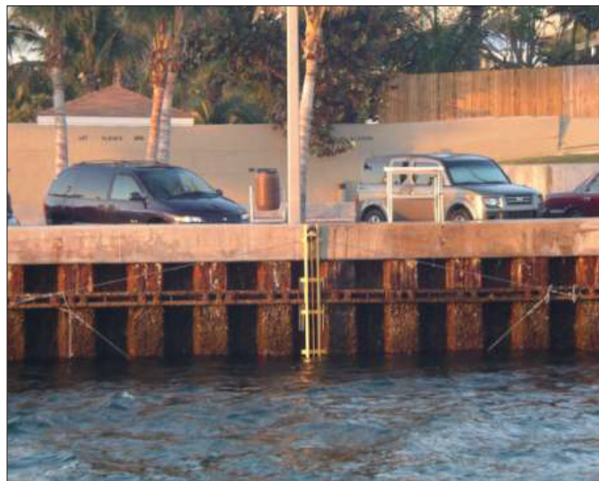
Figure 4. The flow measurement system mounted on the north bulkhead of Boynton Inlet.
